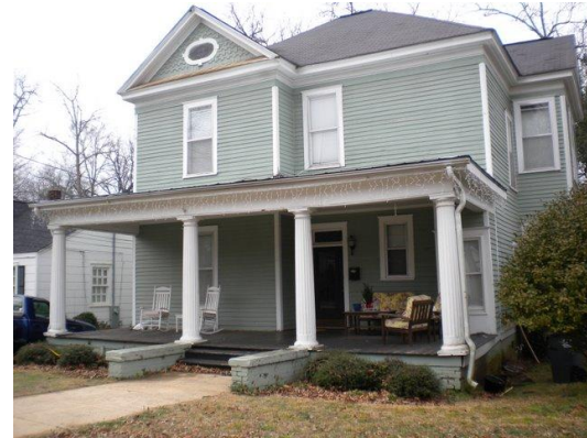
Rating 2: Deteriorated Minor
