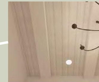
wood ceiling & beams
